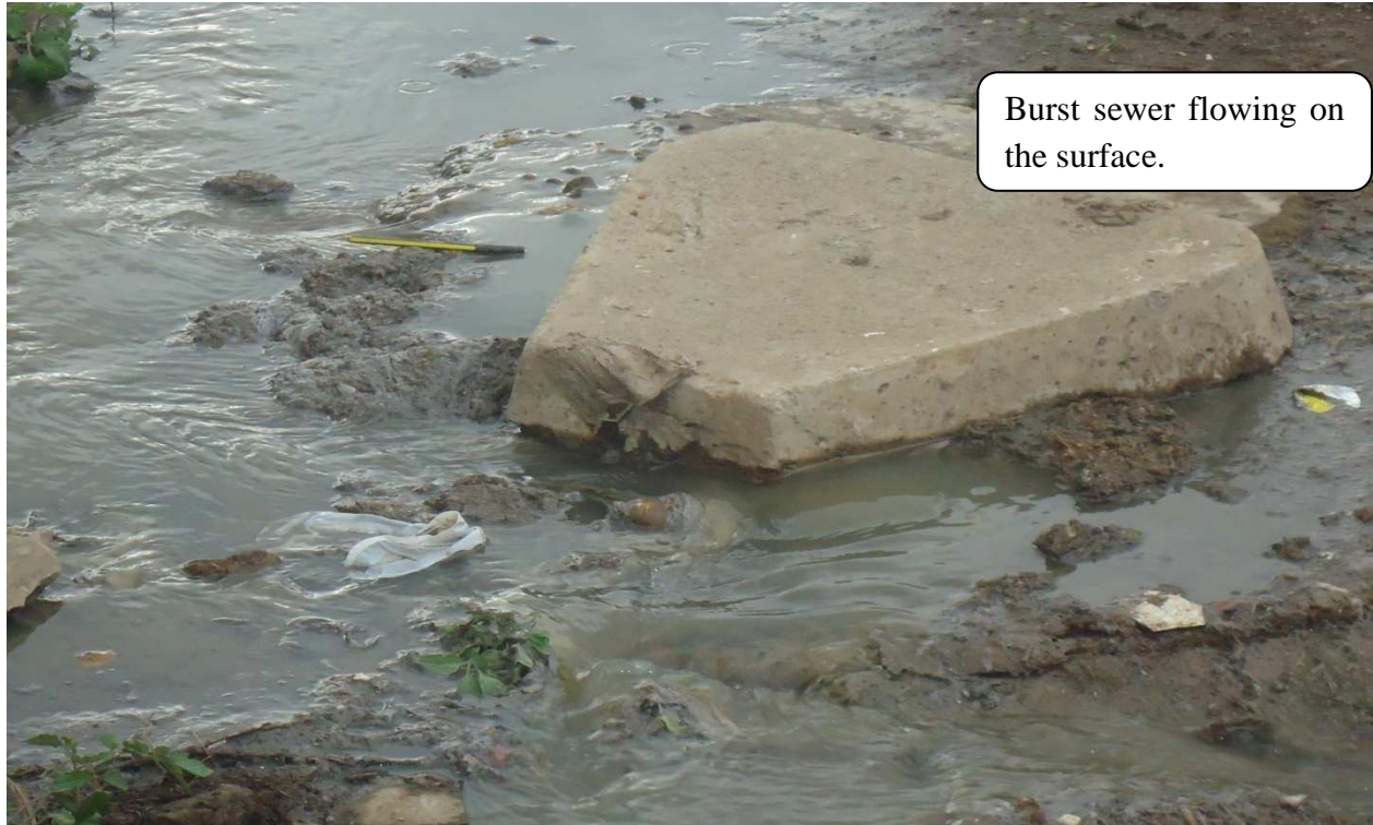
Plate 5.4: Implication of uncontrolled development on pollution (Busted Sewer).
