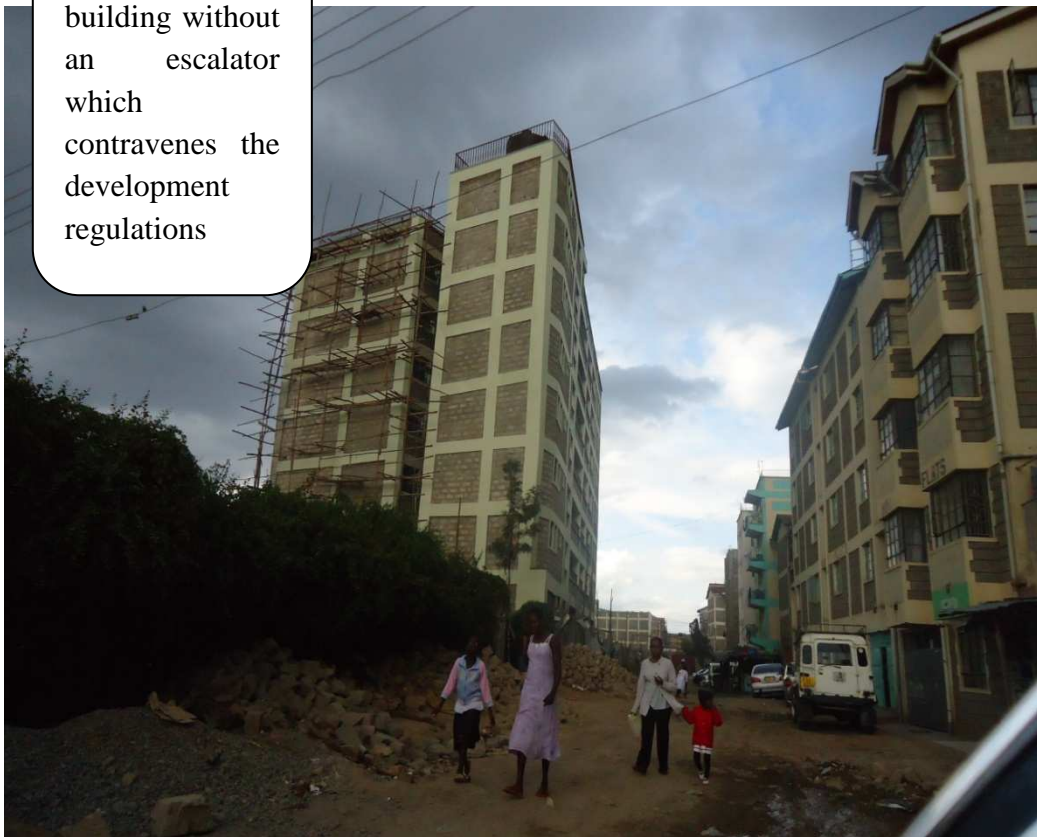
Plate 4. 1: Highrise storey buildings without escalators.
