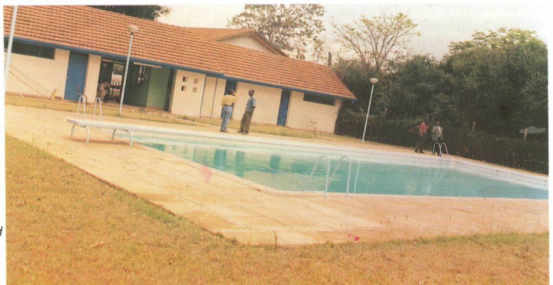
The newly refurbished swimming pool at Parklands Campus
