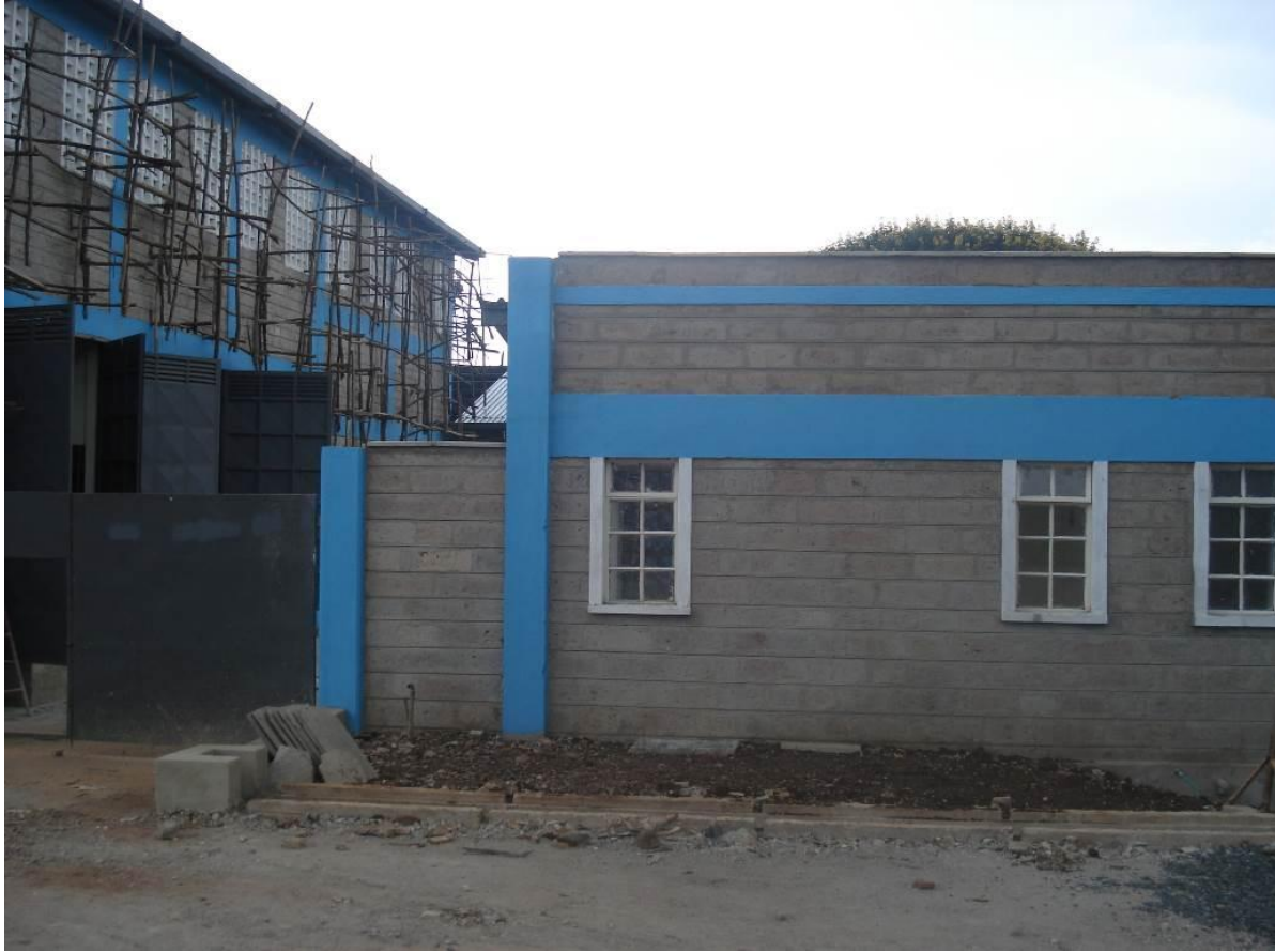
Seed processing Unit under construction at the Field station, CAVS
