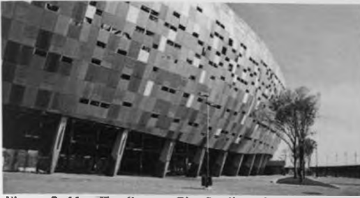
Figure 2. 11 – The Soccer City Stadium façade. Source: Lanxess, 2010.
