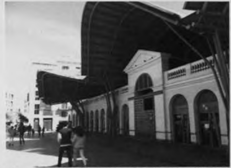
Figure 5.20 – The interesting mixture of the old classical building with the new roofing. Source: Author, 2013.
