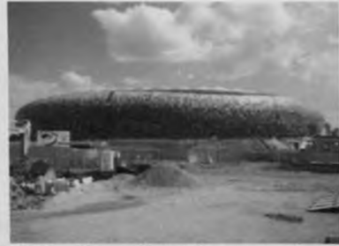
Figure 2. 12 – The stadium under construction. Source: Author, 2009.
