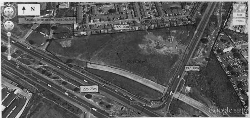
Figure 4. 39 – Site II area and façades. Source: Author based on Google Earth, 2013.
