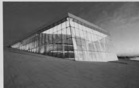
Figure 2. 2 – The sloping roof of the Opera House. Source: Statsbygg, 2005.
