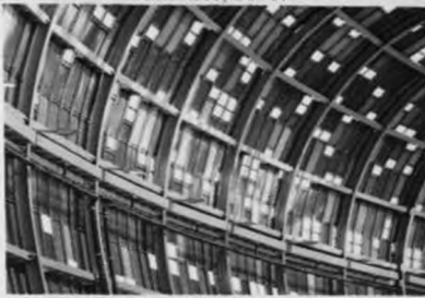
Figure 2. 13 – The glass-fiber concrete wall view from the inside. Source: Lanxess, 2010.
