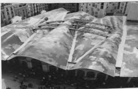
Figure 5. 26 – Saint Catherine Market roof project. Source: Eric Miralles, 2005.
