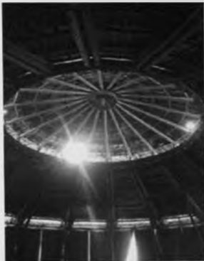
Figure 4.4 – Big Hall's roofing. Source: Author, 2013.
