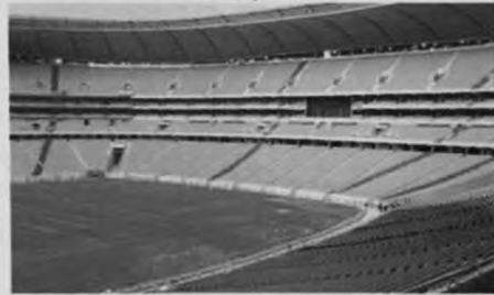
Figure 2. 14 – The Soccer City Stadium internal view. Source: Fujitsu, 2010.
