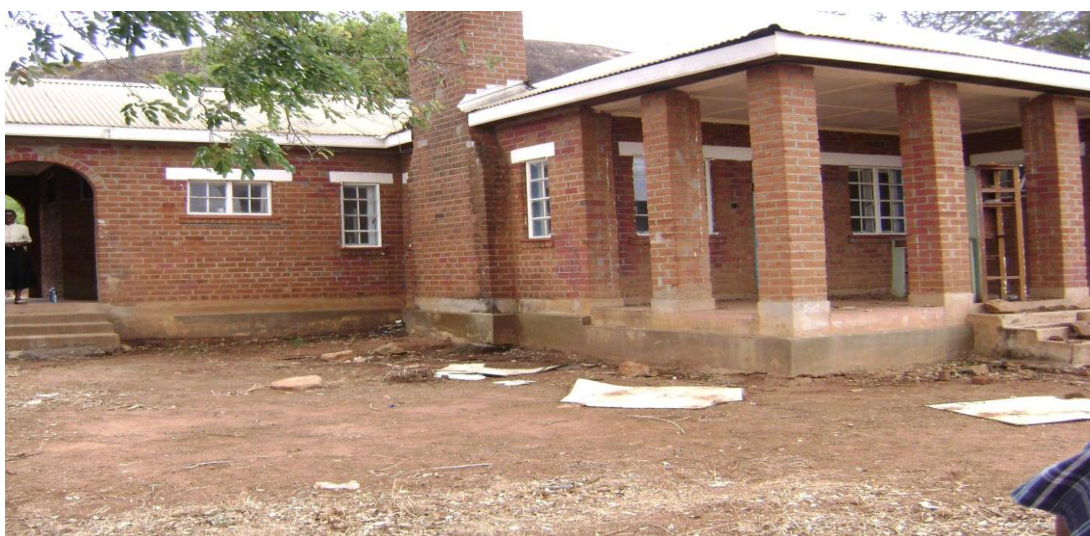
Figure 9: Building to be renovated for Mwingi DICE
