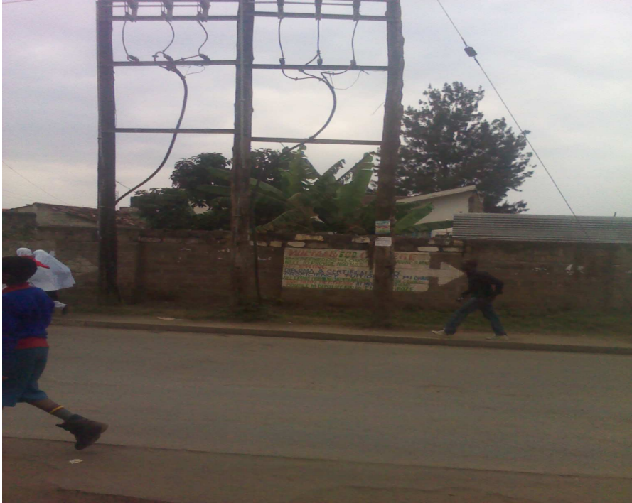
The good road and power networks. At the background are the banana, avocado and grievallia trees within the estate.
