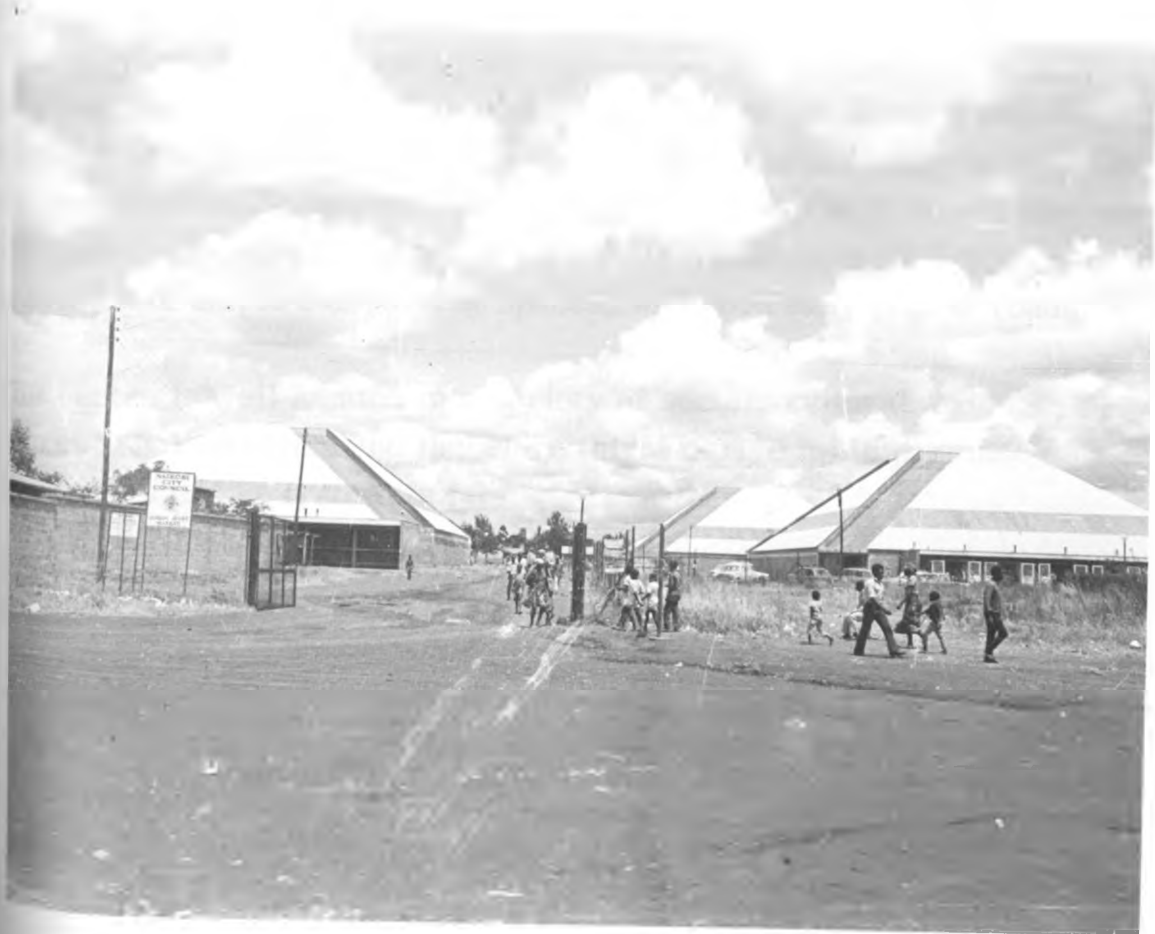
Newly constructed market halls for phase one
