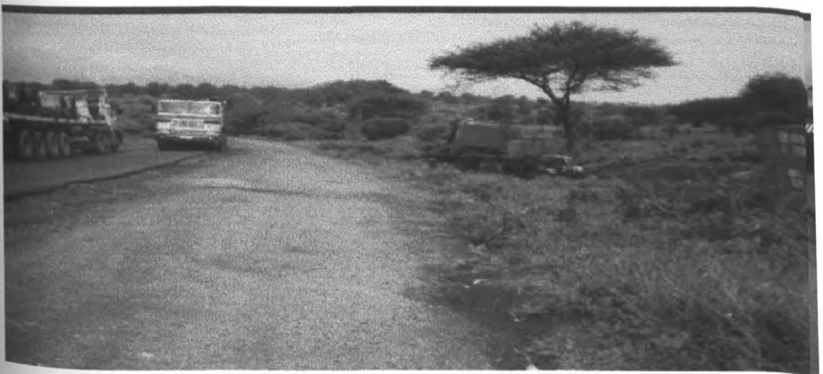
Plate 4. An accident as a result of a narrow road with very steep edges.
