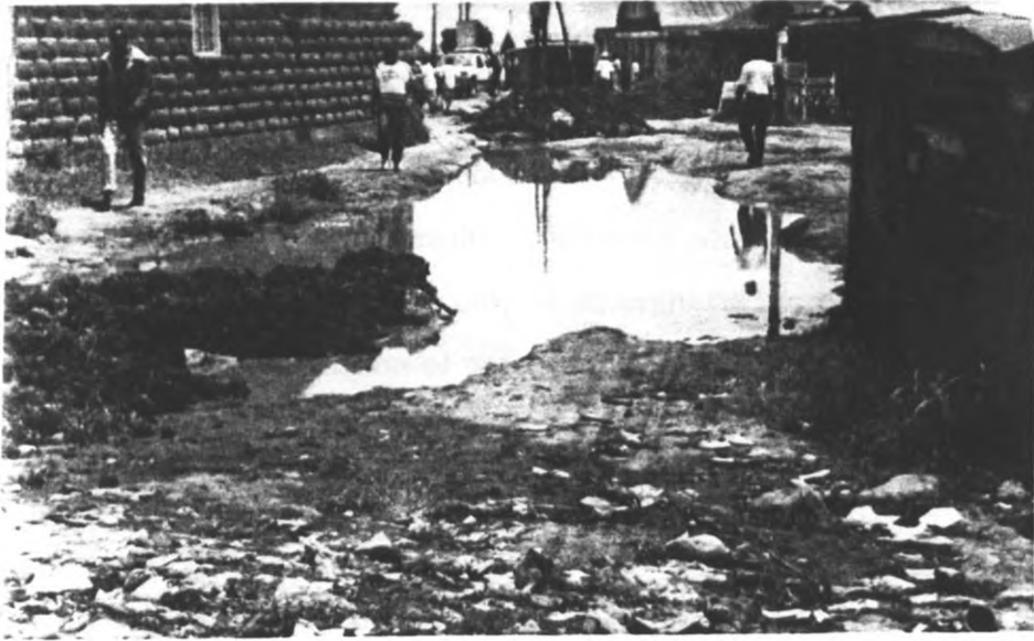
PLATE 5: Harphazard methods of covering depressions present on many streets have made some of the streets immortorable. This has, however, not drained off the waste water pools.
