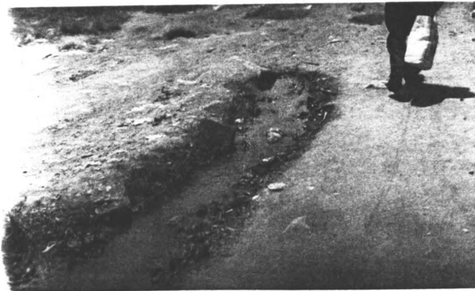
PLATE 8: Some multi-storey blocks do not seem to have any waste water draining from them. The reason behind this is that waste water is drained through underground pipes on to the street
