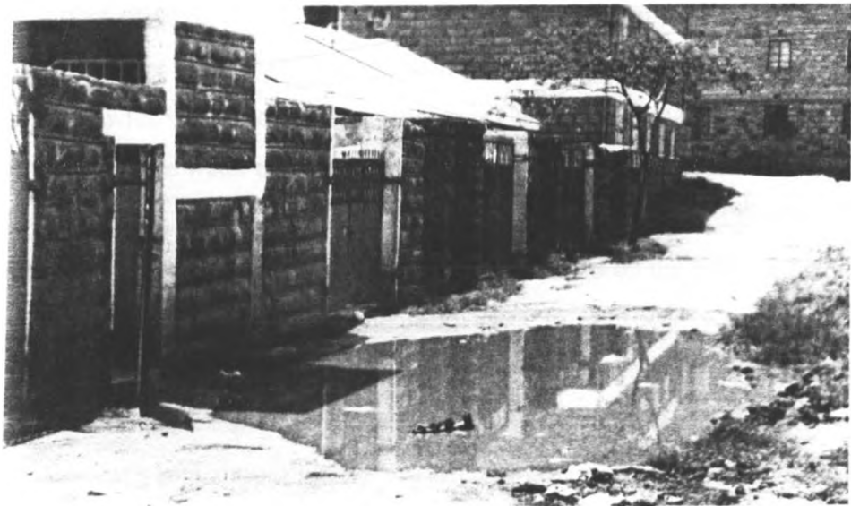
PLATE 6: Along some streets, waste water in form of pools have made it difficult to access the house units through the gate.
