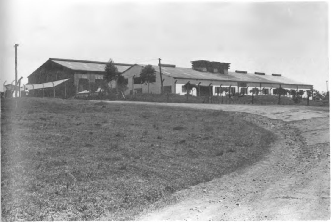
Plate 1 : The Nyansiongo Tea Factory.
