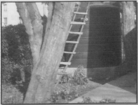
Plate 48: Water tank at Iko toilet
