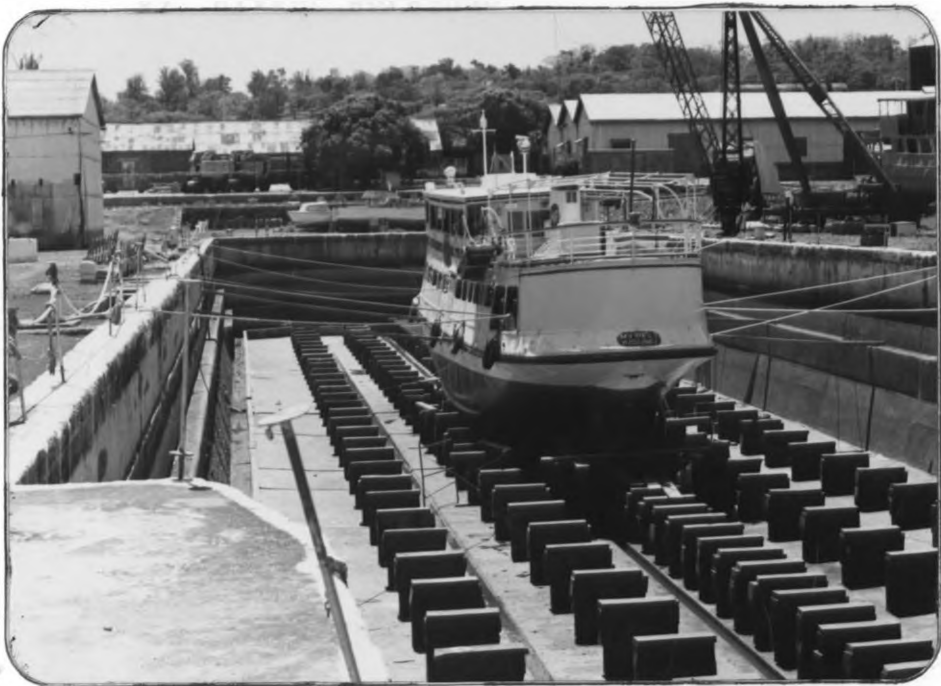
PLATE 5: M.V. RELI AT THE DRY DOCK
