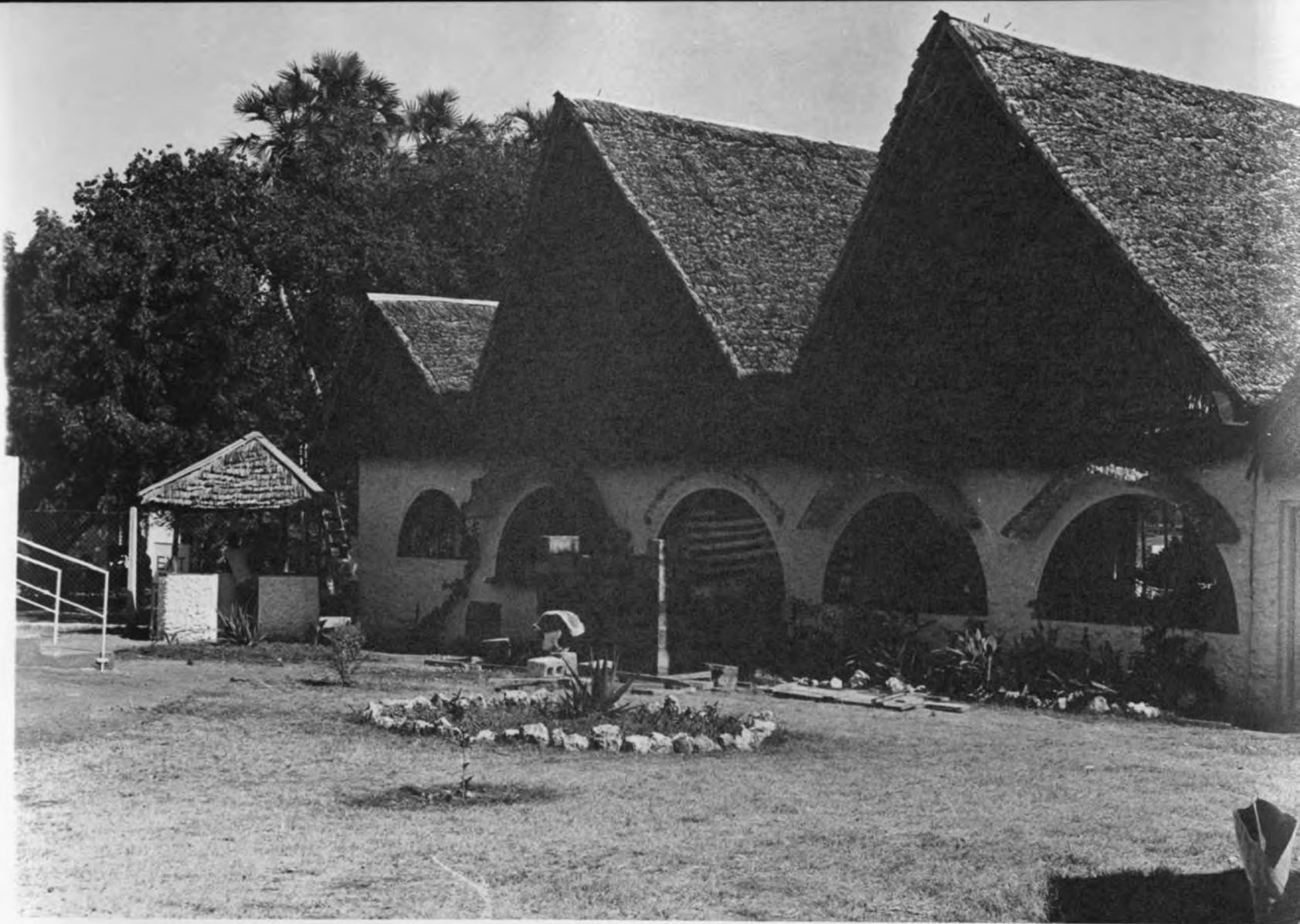
THE LOUNGE-BAR AND THE TICKET BOOTH. NOTE THE ADDITIONAL TANK UNDER CONSTRUCTION
