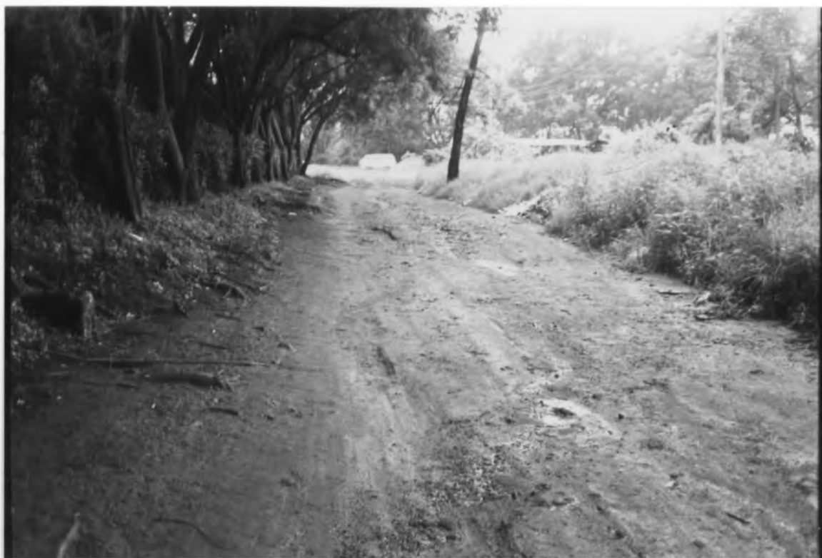
Plate 5: Some of the prevailing road conditions in residential areas. The lucerne crop on the unfenced roadside plot covers part of the road.
