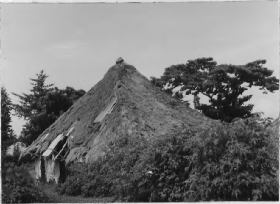
Plate 4-8: A Poorly maintained Kisii thatched house.
