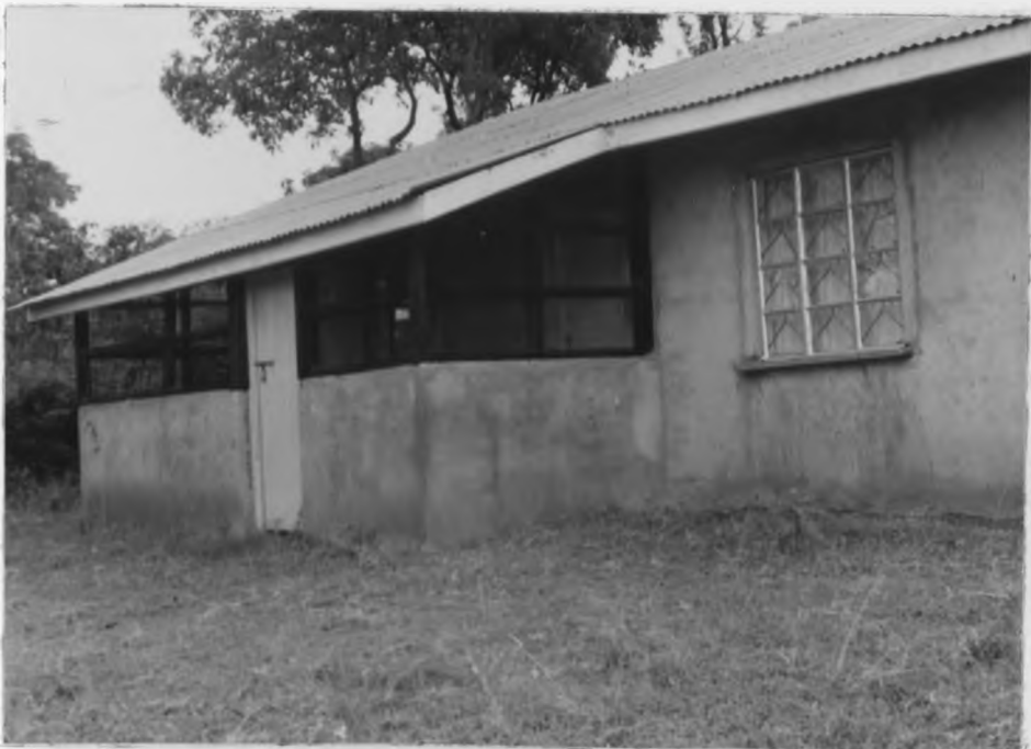
Plate 4-5: A Block Permanent House.
