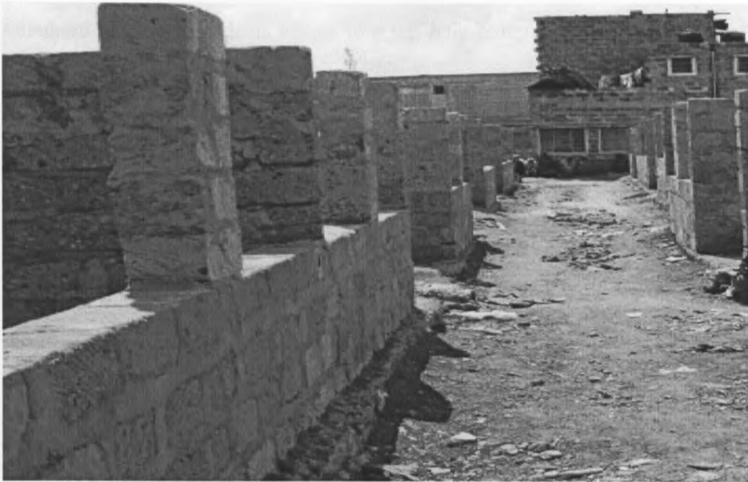
Plate 5.1 Houses under construction in Mahira informal settlement
