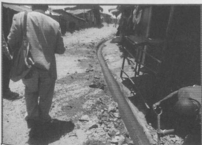
Cleaning of the drains. Source: Field Survey, 2012
