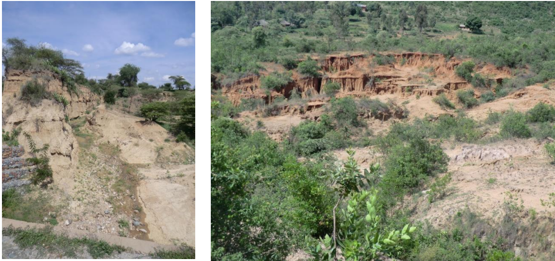
Figure 1 2. Soil erosion documented during field studies in the Lower Nyando
