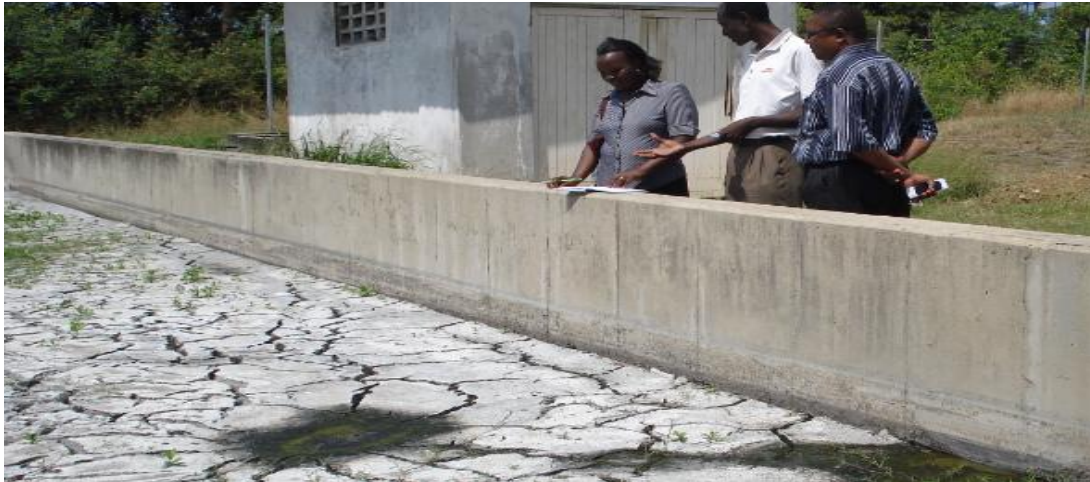
Figure 2.6: Twenty one sludge drying beds
