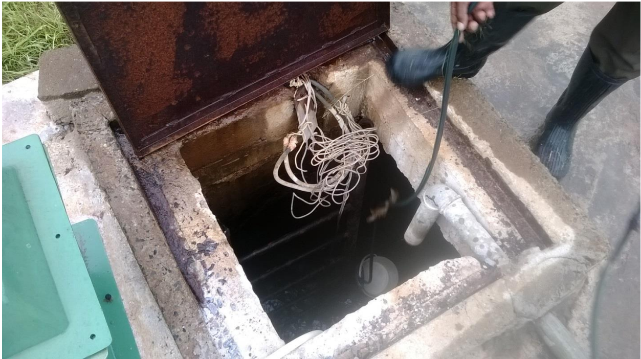
Plate 6: Oloolaiser Water Treatment Plant Clear Water Tank.
