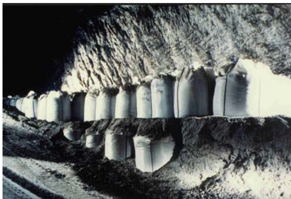
FIG. 3. Refilling with large bags
