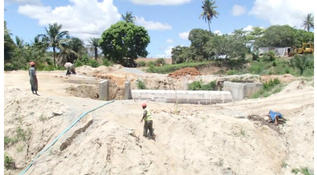
Figure 7-20 Weir Intake Under Construction
