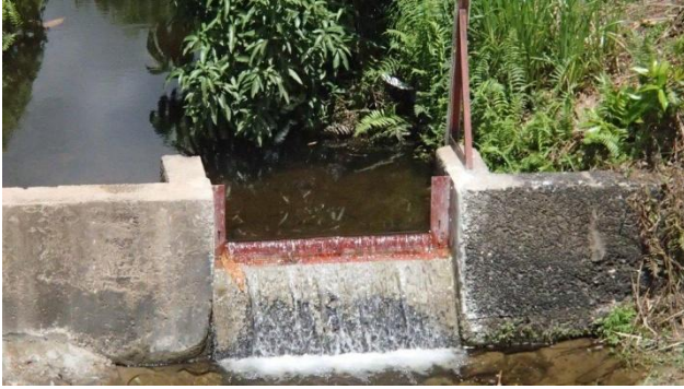
Figure 7-3 Repaired 3KD06 River Gauging Station
