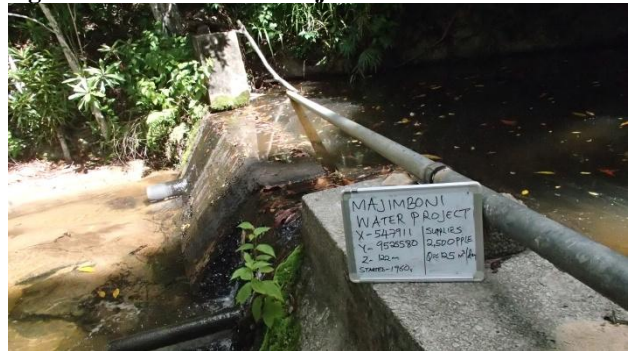
Figure 7-26 Intake for a Water project
