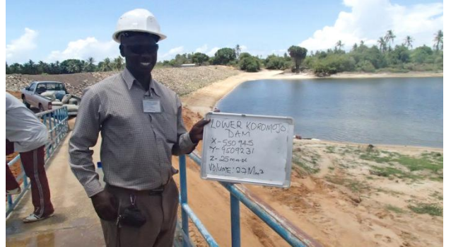
Figure 7-24 Lower Koromojo Dam
