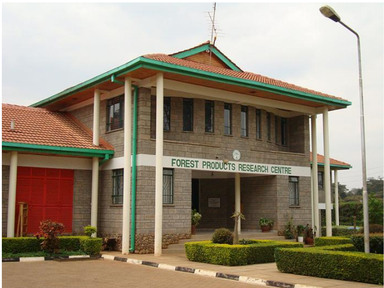
Plate 1: New KEFRI building at Muguga.
