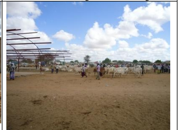
Picture from a follow-up visit showing new sheds under construction.
