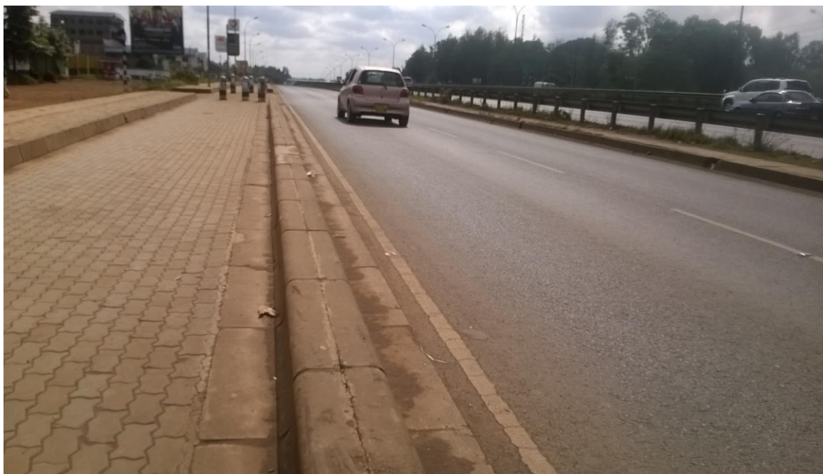
Plate 19: Raised Kerbs along Thika Super Highway at Safari Park Hotel
