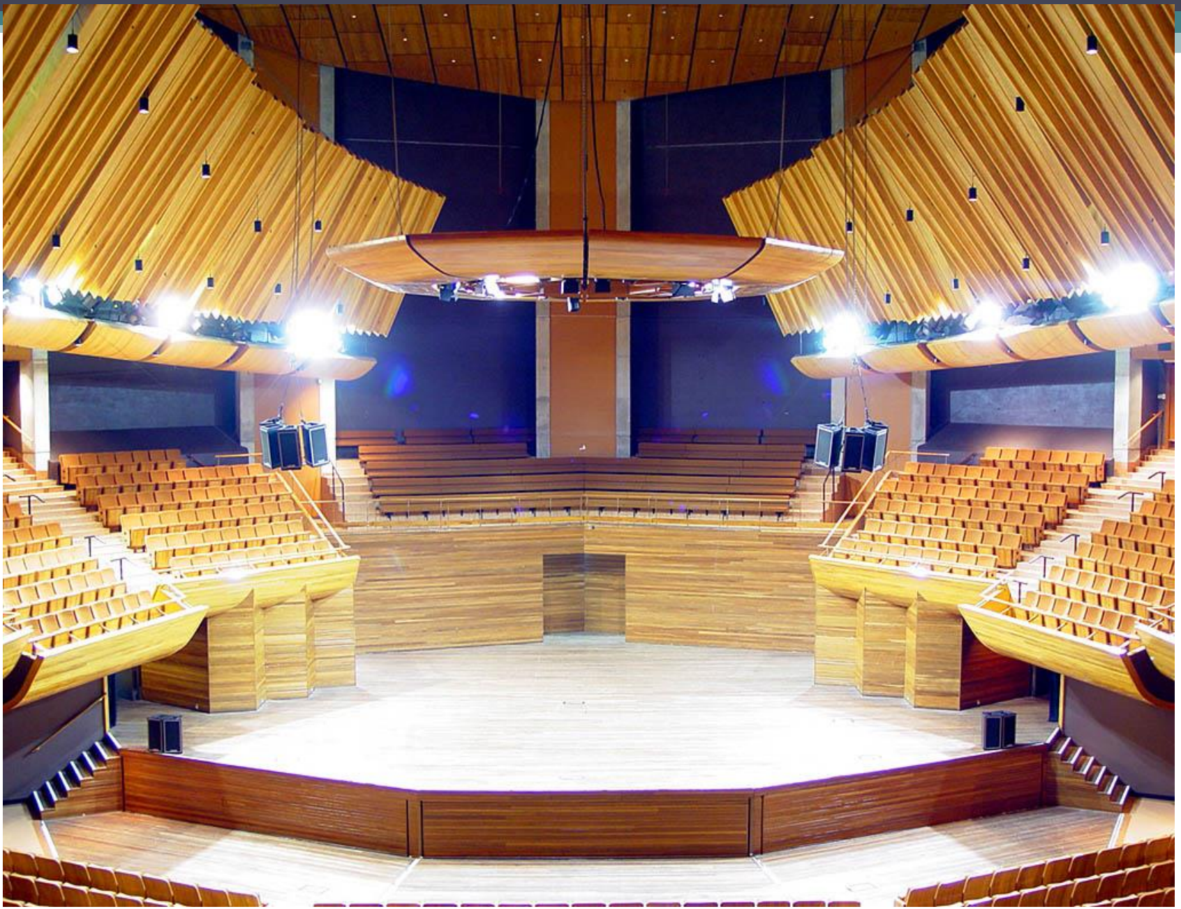
Hall with a raised stage and curved acoustical reflectors above the stage
