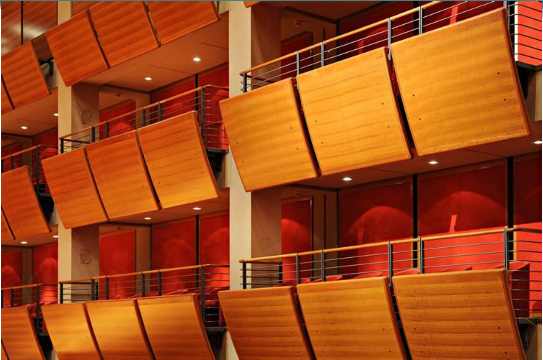
Auditorium del Lingotto Torino, Italy. Detail of the curved balcony sound reflectors
