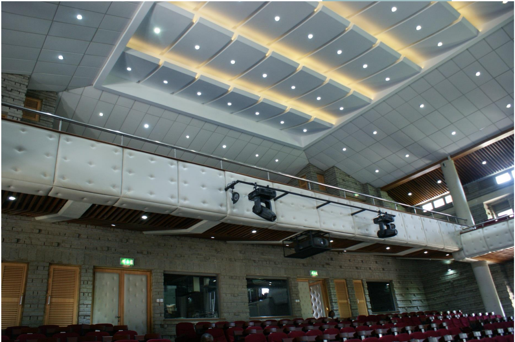
Acoustic ceiling and sound absorbent vinyl covered balcony beams
