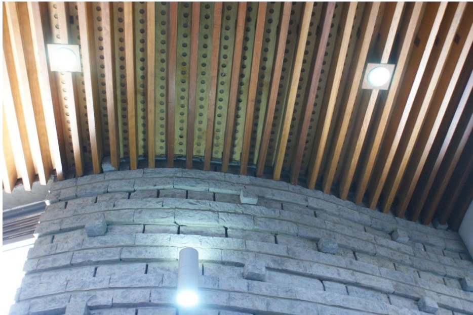
Timber joists acoustic ceiling
