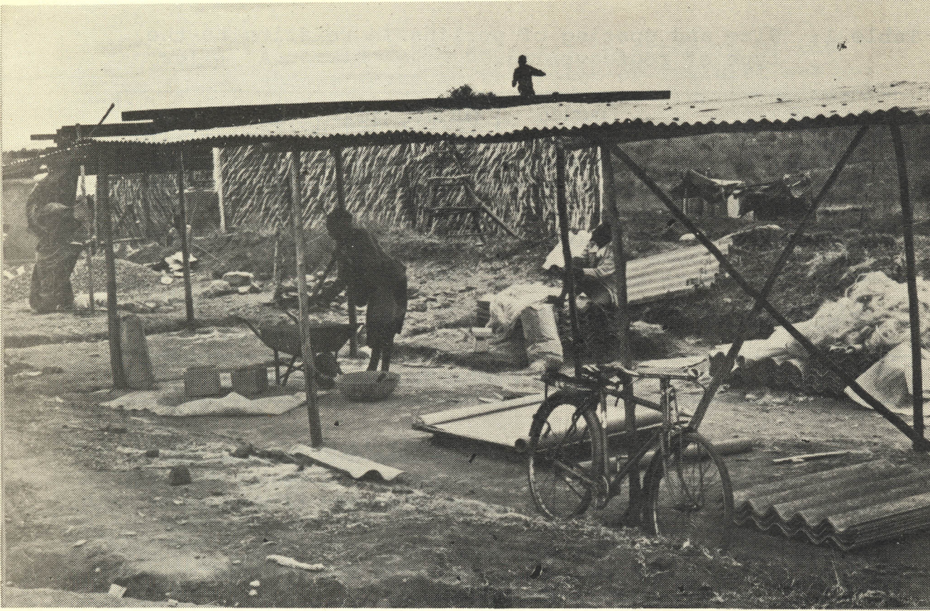
5. The production place for the roof sheets
