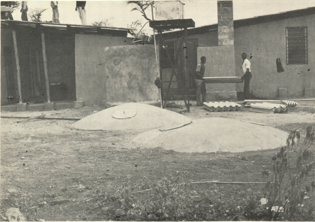
41. Overview of the water storage system.
