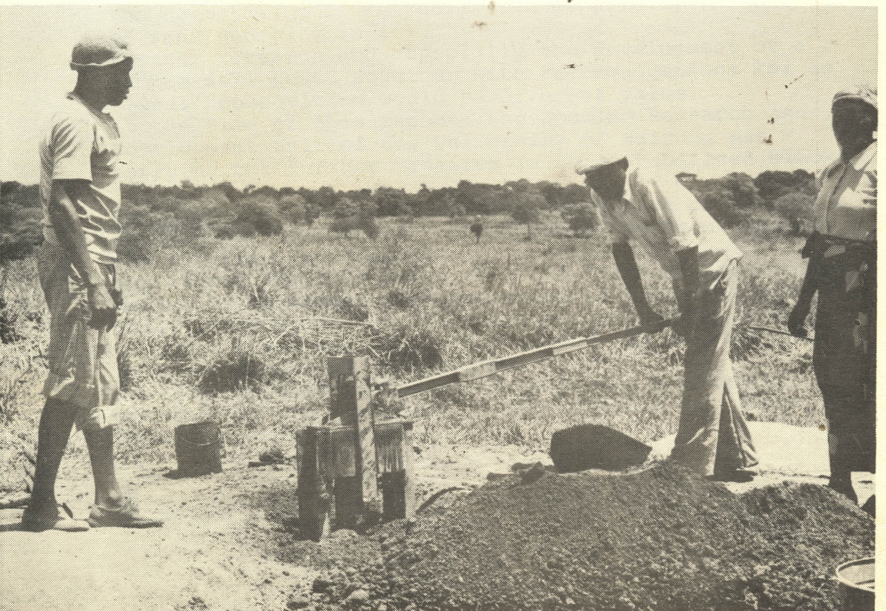
34. The mud-block press, in compression position
