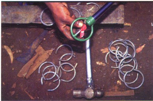
PHOTO 35: SHAPING THE CIRCULAR FRAME
