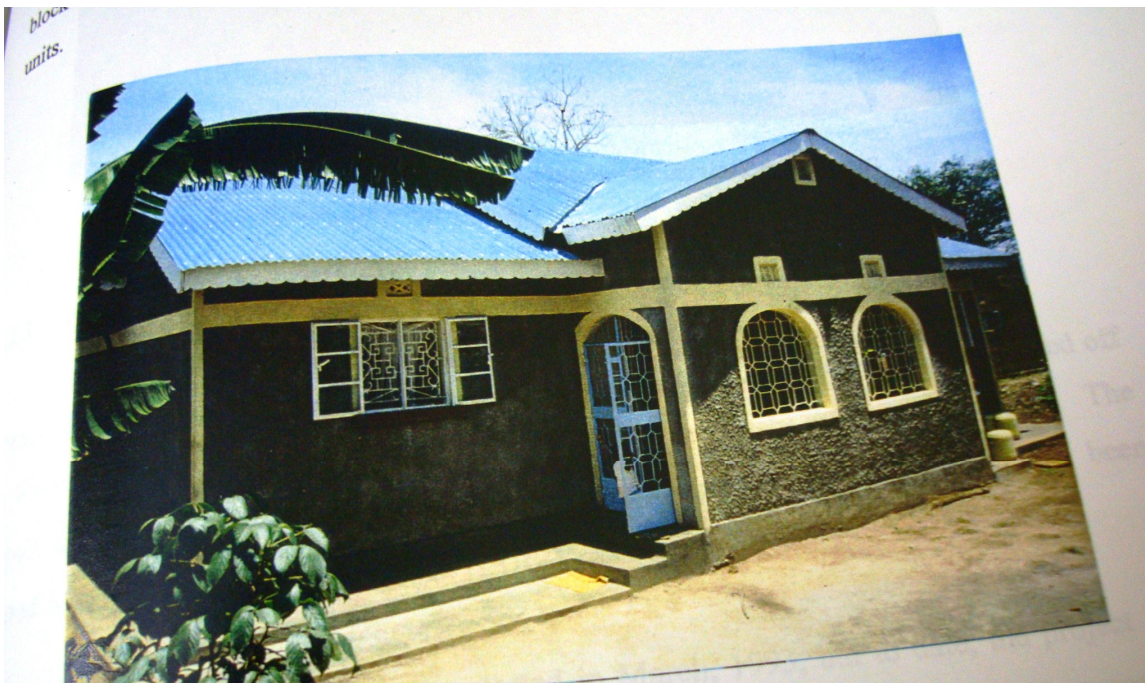
Fig. 3.4: SSB Rental Houses at Marachi Estate with GCI roof - Expansion of Technology
