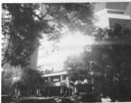
Fig. 6.3: Glare emanating from building's facade Source: Field survey, 2012 -KEMU Towers glare in CBD Nairobi creating discomfort to pedestrian using side walks
