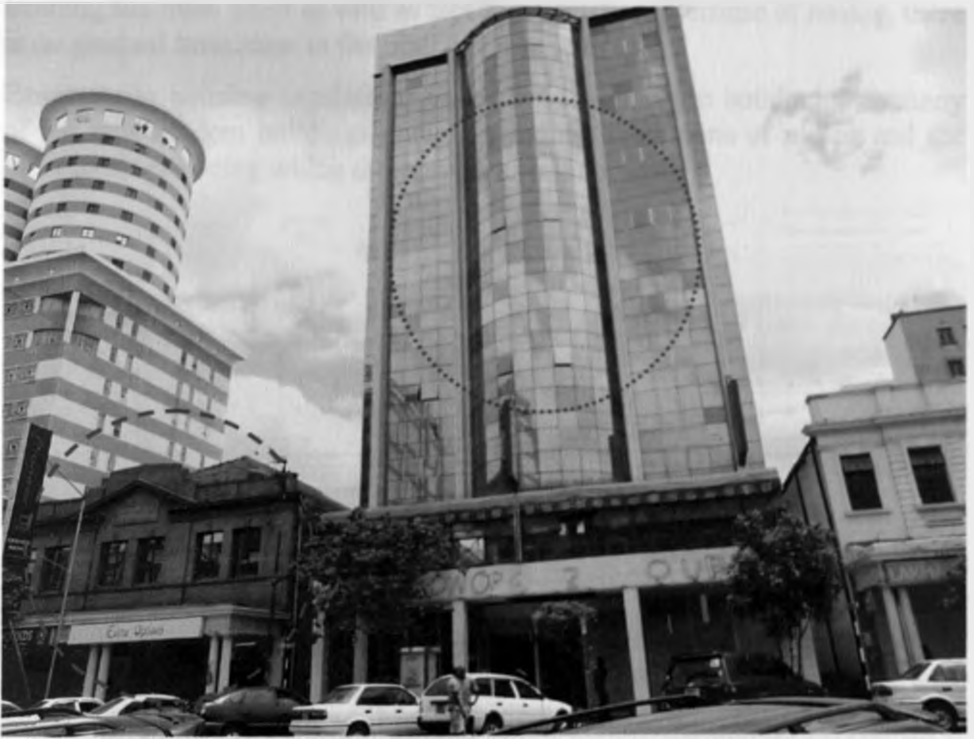
Fig. 5.18: The 1930's Art-Deco buildings and the Modern glass-clad Source: Field Survey, 2012
