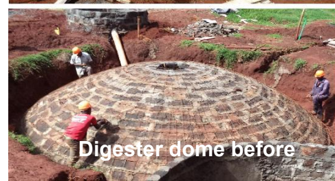
Digester construction at 2nd ring
