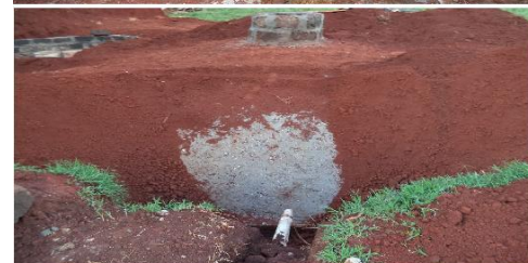
Digester dome after
