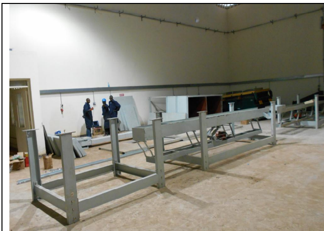
Laying of frames at onset of installation process
