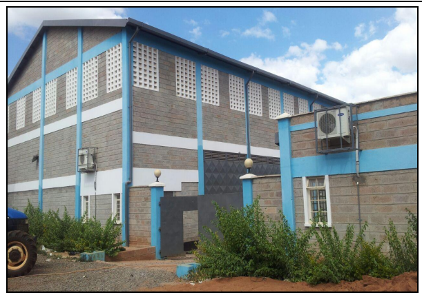
Completed factory building where the processing machines are housed
