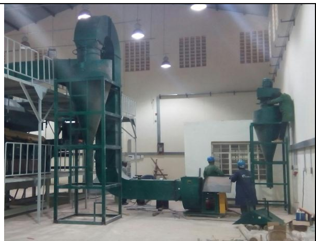
Duct extension works for air screen cleaner cyclone
