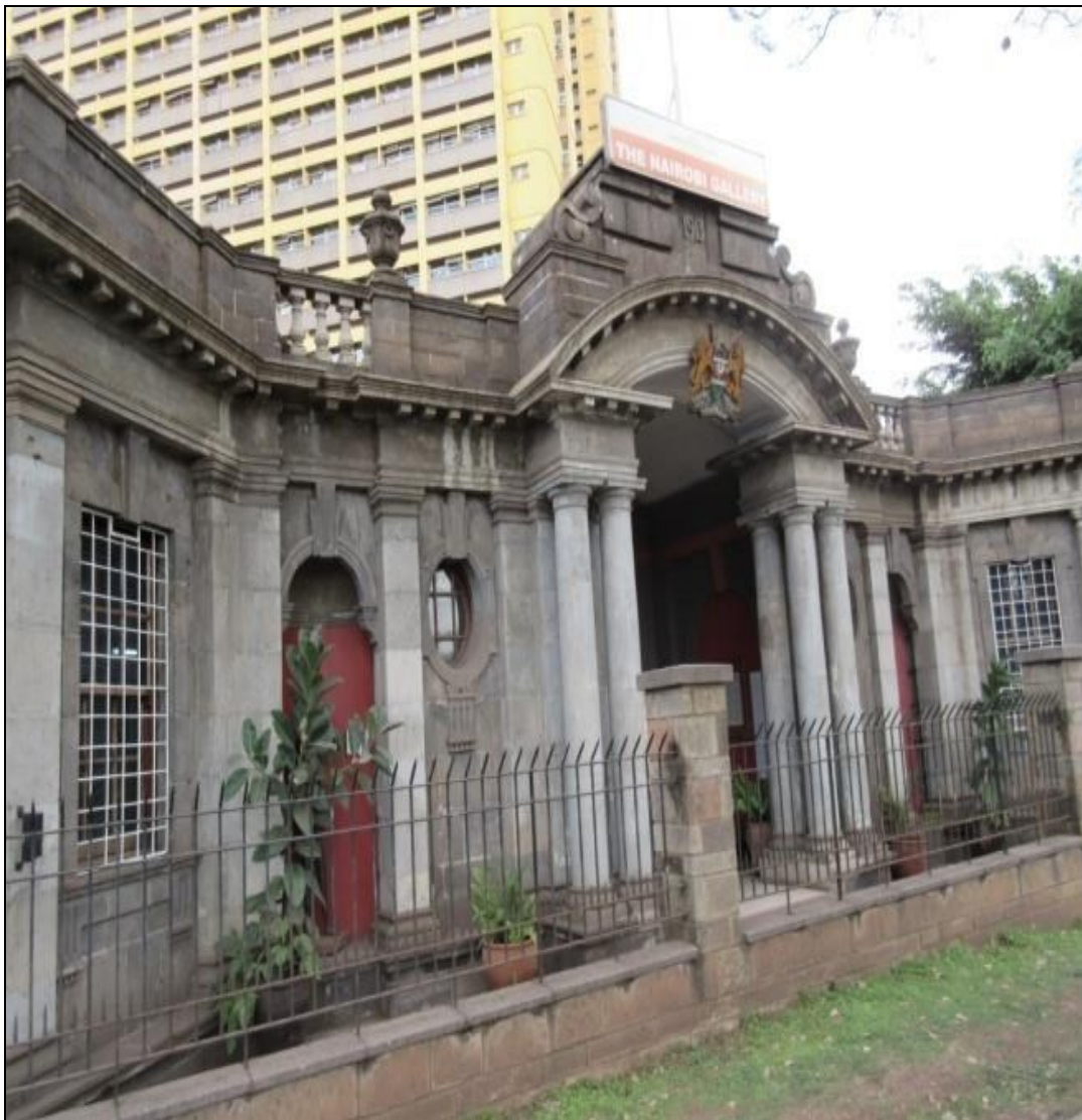
Plate 4: Facade of Old Nyayo House.
