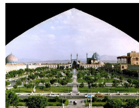
Fig 15. Imam square. Isfahan, Iran, showing the pure traditional Islamic architecture (source: http://pinterest.com )
