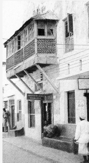
Fig 19. House and shop building with a balcony (source: conservation of Lamu, National Museum of Kenya)
