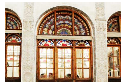
Fig7. A house in Kashan, Iran, showing the use of colorful windows. For beauty and prevention of sun glare. (source: http://pinterest.com )
