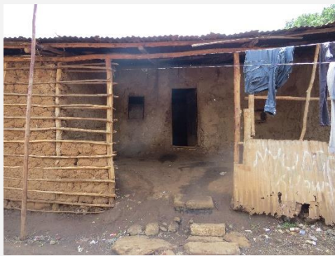
Fig 109. one of the oldest houses in Makina settlement (source: Author photography)
