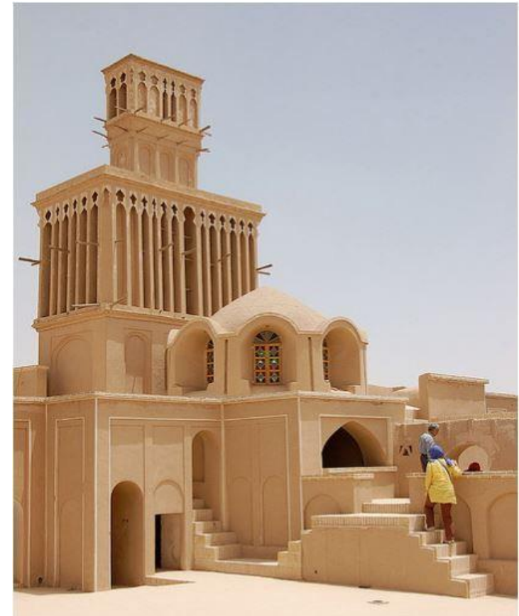
Fig6. Wind catcher in Yazd, Iran (source: http://issuu.com )
