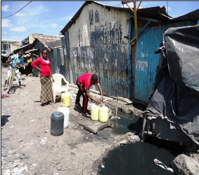
Figure 26 Plate showing a water vendor serving a customer from a pipe running under sewer water (Field study, 2014)
