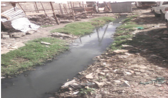
Plate 4.14 Poor drainage system with open sewer photograph
