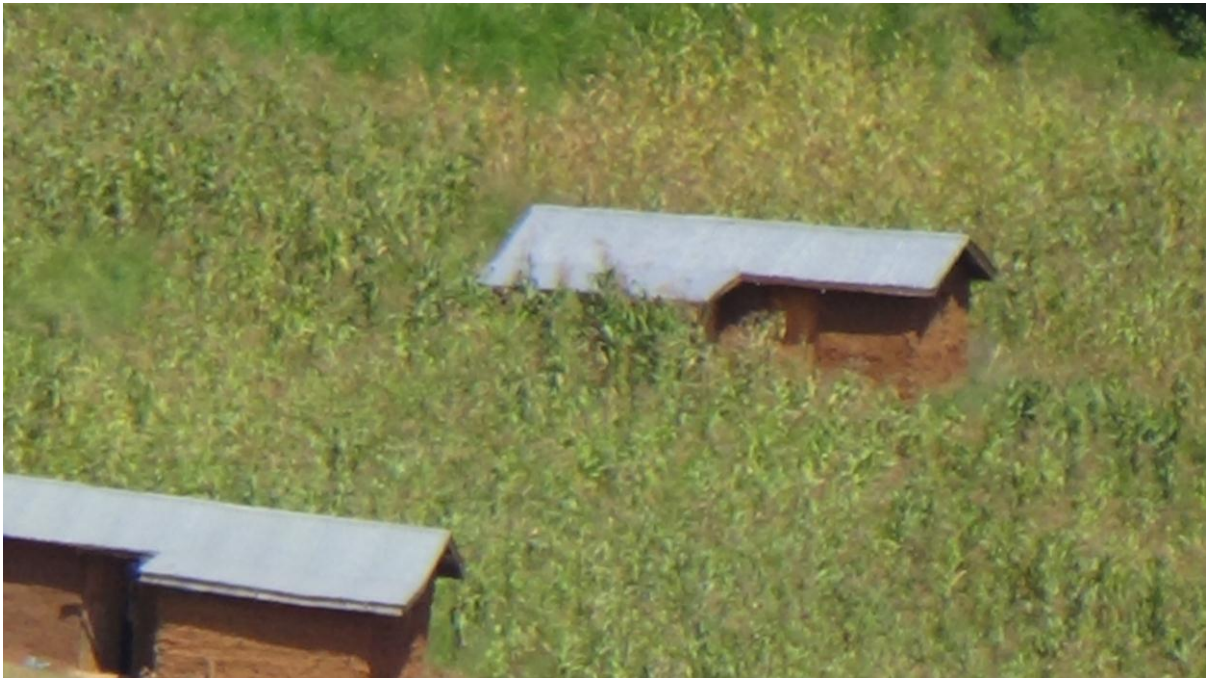
Plate 9: Some of the rebuilt but un-occupied houses in Metta village
