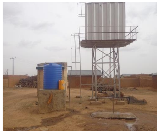
Plate 5.39: A functioning Motorised Borehole in Maigora Community, Maintained through Toll (Pay-Per-Fetch) Collection System
