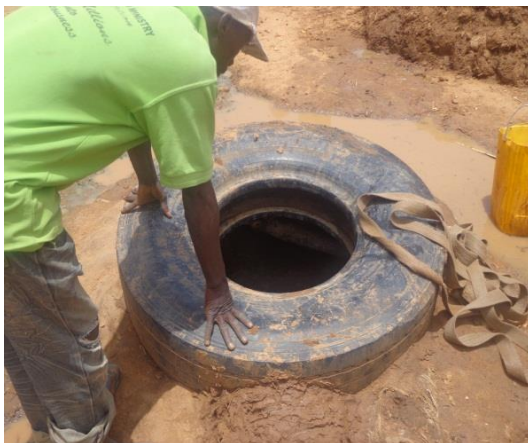
Plate 5.44: Using an Old Vehicle Tyre to Gauge the Mouth of an Open Well to Prevent it from Widening at Tudun Jae Community, Danja LGA
