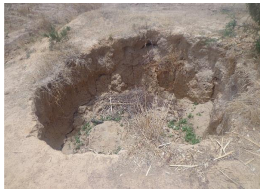
Plate 5.33: An Ordinary Open Well Abandoned due to Collapse of its Sides at Mallamawa Community, Matazu LGA.
