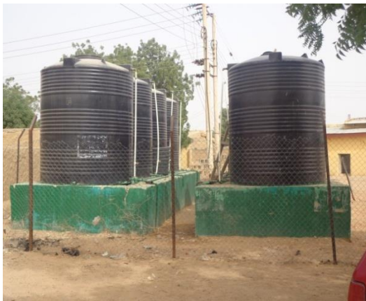
Plate 5.46: Plastic Water Tanks Provided at Walawa Community in Kaita LGA to help Store Water Supplied to the Community using Water Tanker
