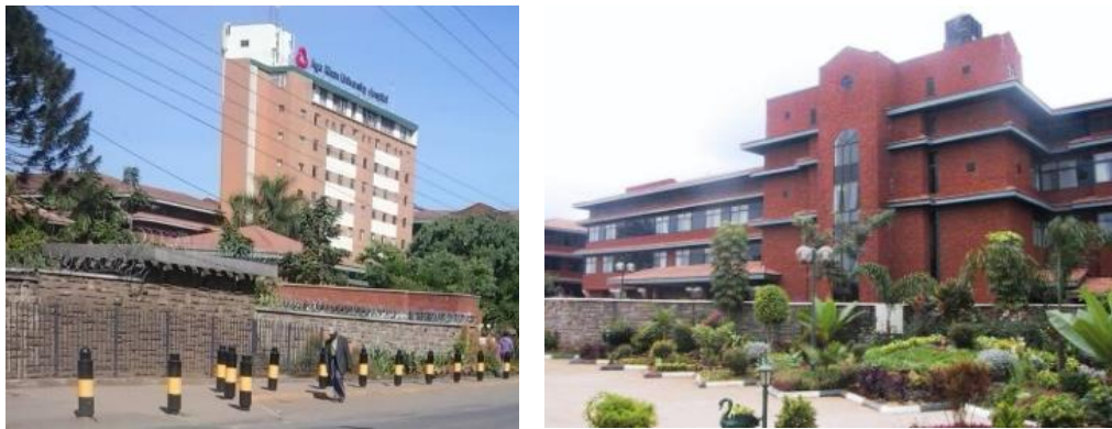
Figure 5:23 various buildings in the Aga Khan University Hospital, Nairobi
