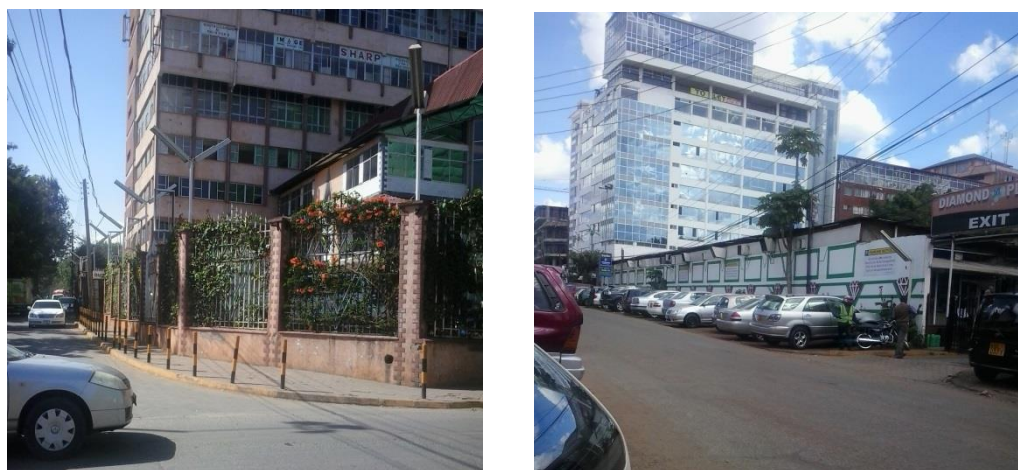
Figure 5:16 Treatment of the edges of the commercial block along Mutati, Masari Road and Fourth Avenue respectively.
