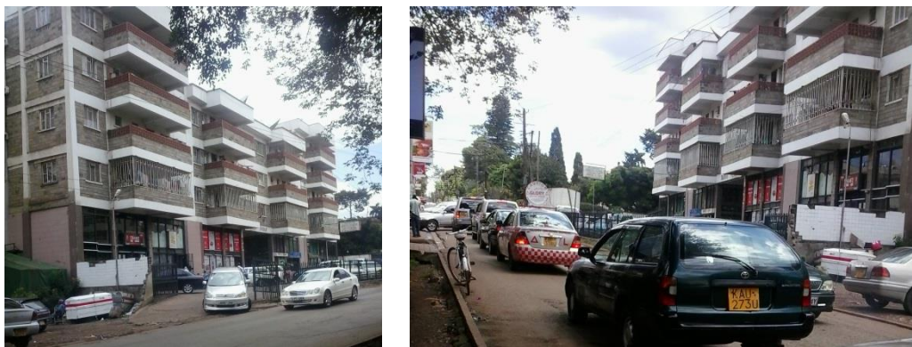
Figure 5:21 Deep balconies on the facade of Amani Plaza
