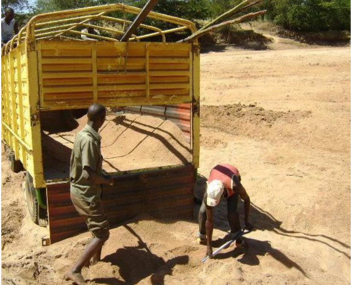
Figure 3-2: Workers collecting sand for construction
