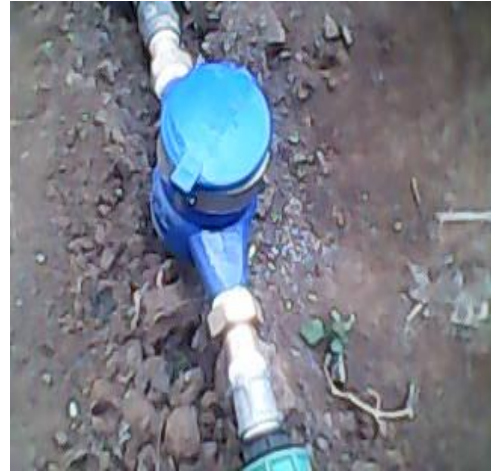
Figure 3.6: Installed water meter
