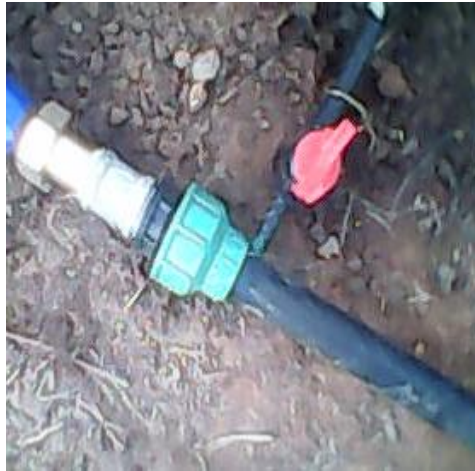
Figure 3.5: A Fitted mini-valve
