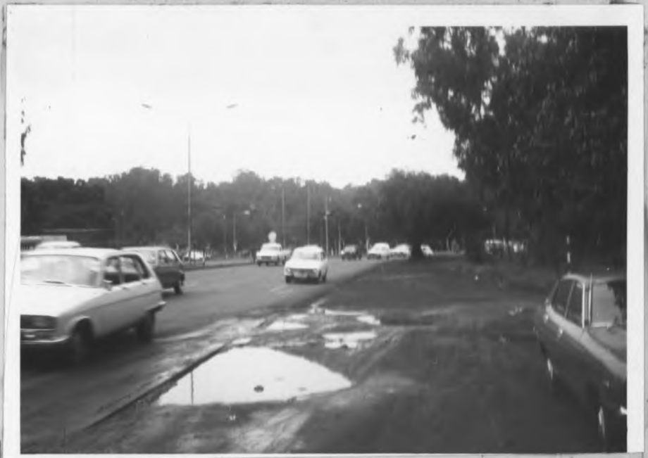
PLATE 11. In search of parking space, motorists break road pavement.
