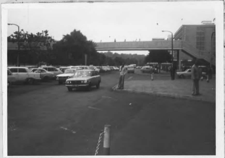
PLATE 15. Pedestrian facilities where provided are under utilized.
