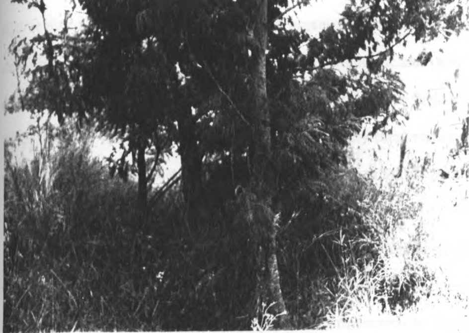
Plate 8: A poorly maintained section of Aguthi canal
