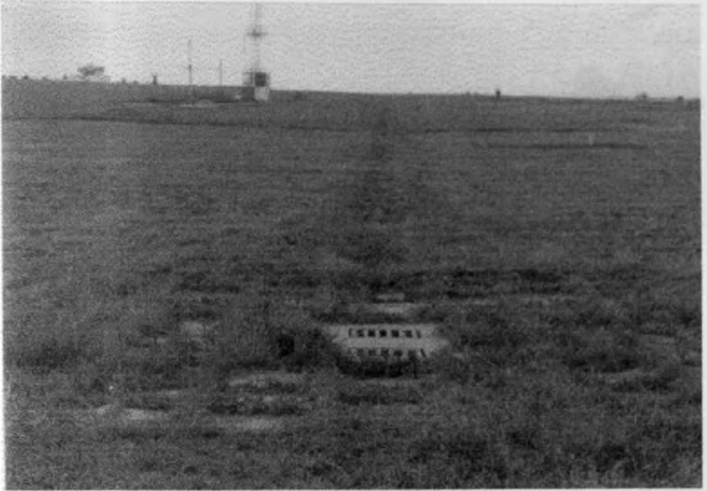
Plate A4.3 Low points of subsoil drain
