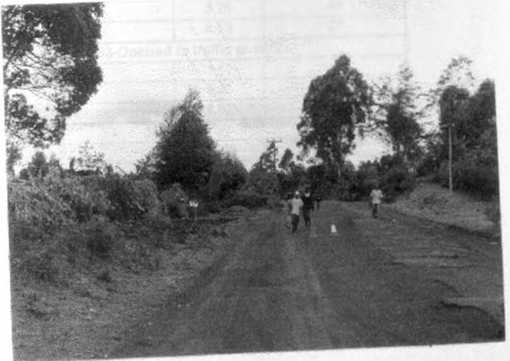
Plate A5.2 Surfacing worn out at ES10 after the 1997/98 El Nino rains
