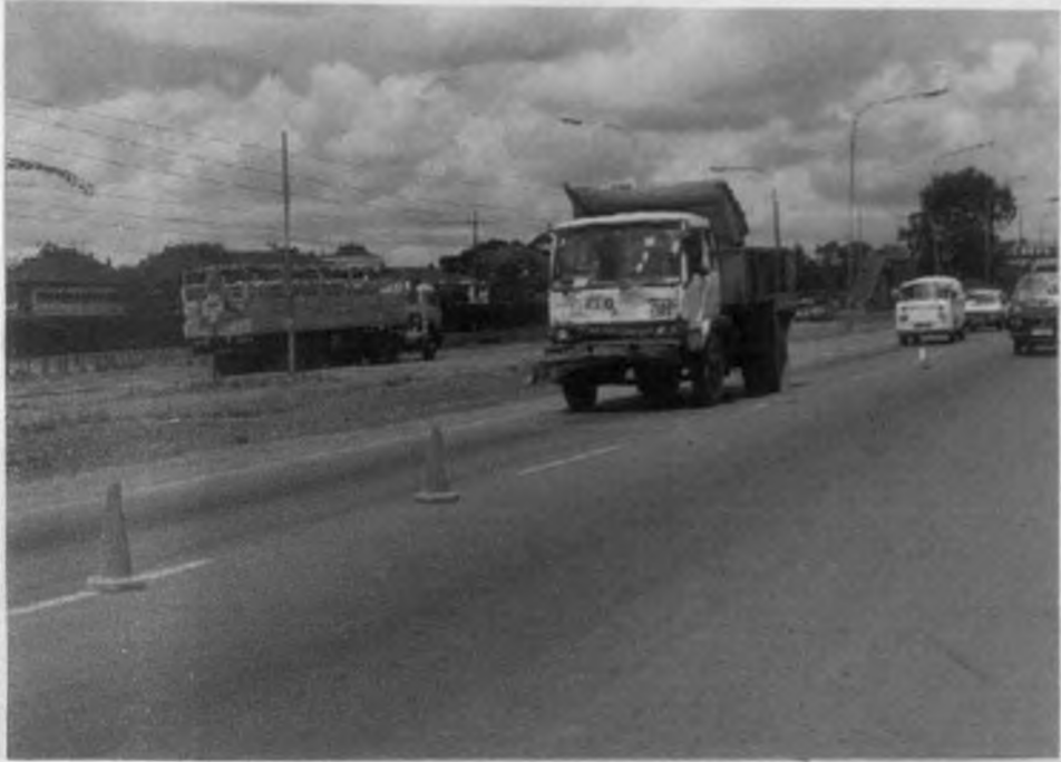
Plate A3.7 Test site ES1 after an overlay
