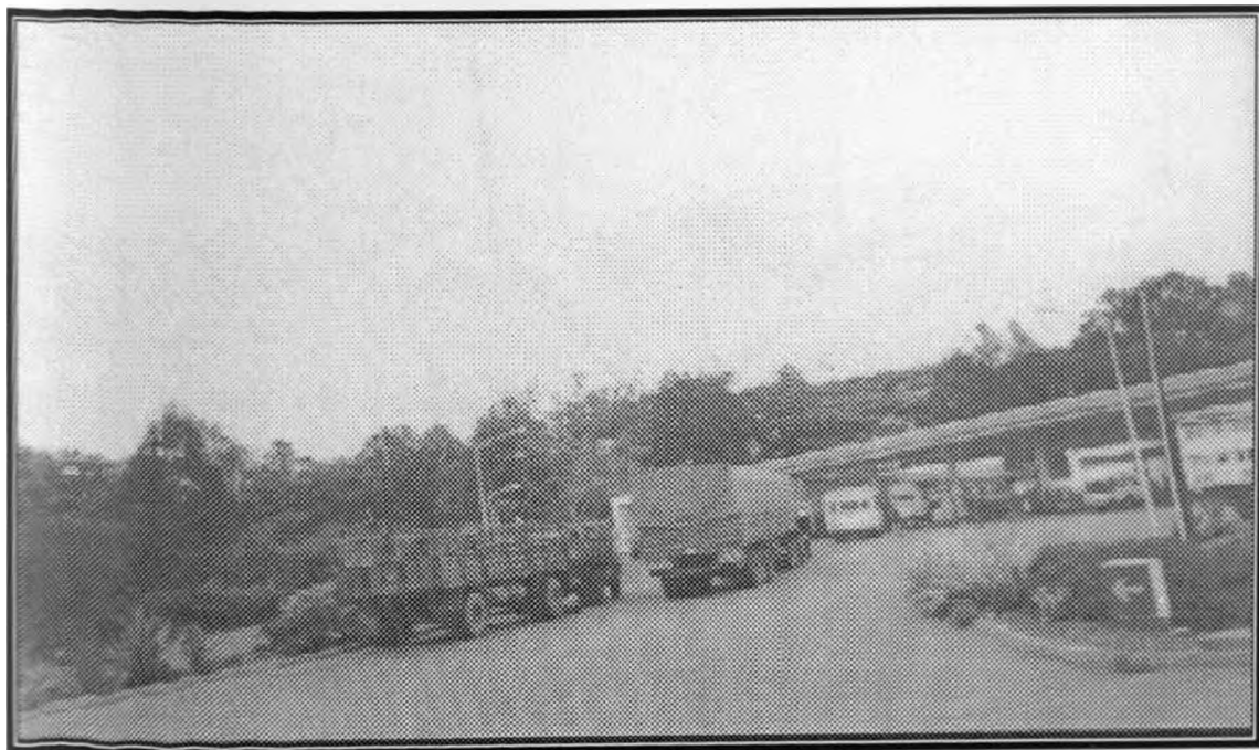
Plate 5.9: Vehicles Parked along Deceleration Lane
