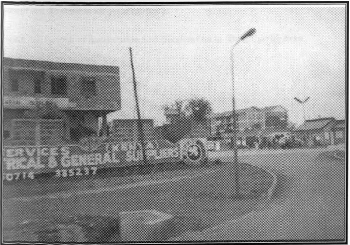
Plate 5.11: A Service Station Without a Well Deceleration Lane
