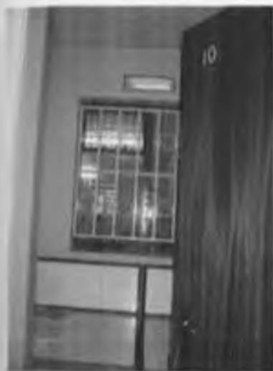
Lighting in carrels, there is dim light due to ageing of the bulb, Source; ibid.
