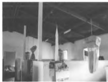
Figure 14: Roof in the male hostel
