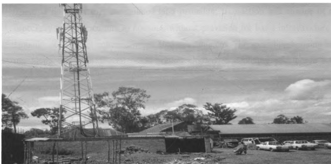
Plate 10: Newly constructed receiver on a newly acquired site.
