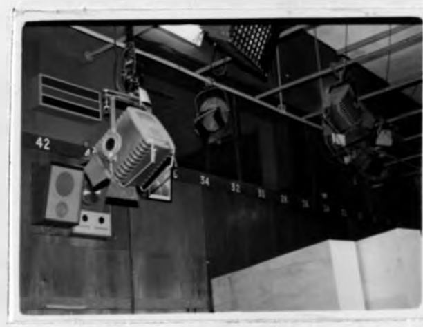
Plate 3.2 Studio Interior showing Control Gallery Observation windows, studio luminaires and the lighting steel scaffold grid. Also note the variation of acoustic materials on the walls.
