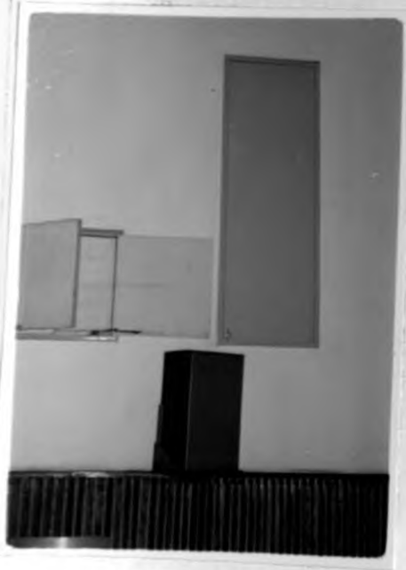
Plate 4.1 Use of Sound Reinforcing System Also note the variable acoustic absorption Panels in both closed and open position.
