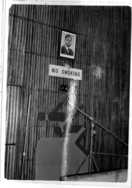
Plate 4.6 Photo showing the nature of the stage wall. Note the hard wood timber strips.
