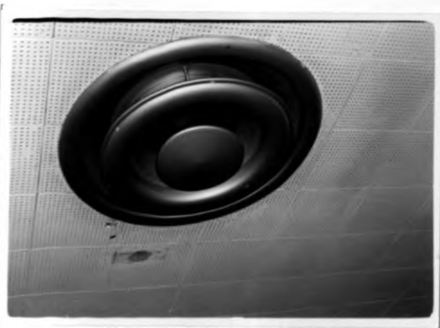
Plate 4.5 Inflow/Outflow air diffuser.
