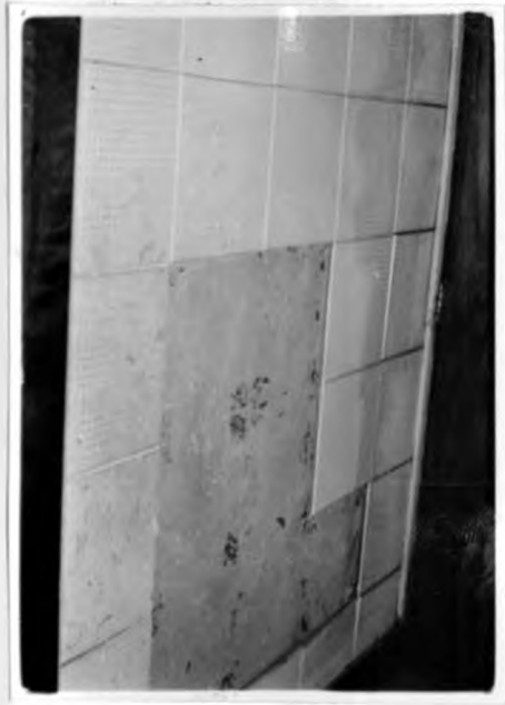
Plate 3,7 Performers' entrance sound lock Note the mutilated acoustic tiles.
