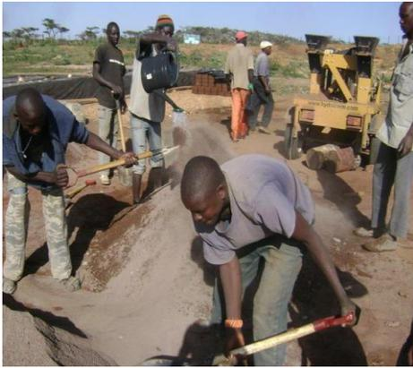
*Figure 3, Mixing of soil and stabilizers*
